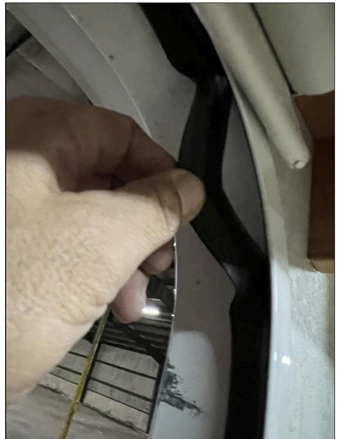
(2) Upper left and right seal of the door frame is coming detached.
