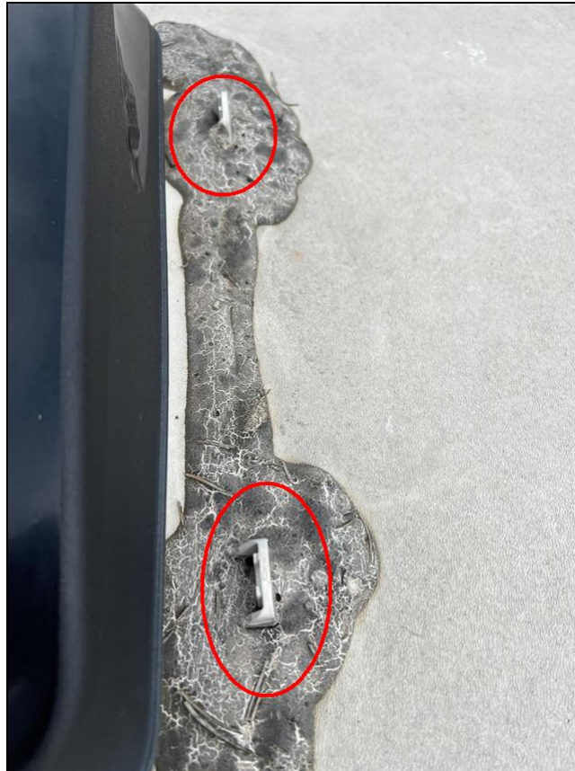
(2) Sealant was not placed in right area around vent.
